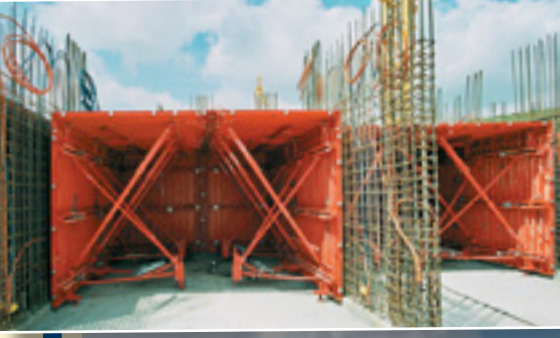
Tunnel formwork system
